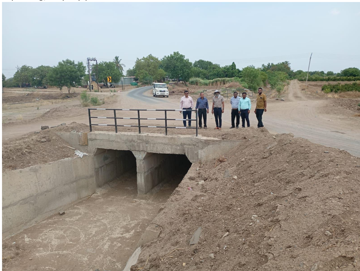
VRB at km 83.342 completed
