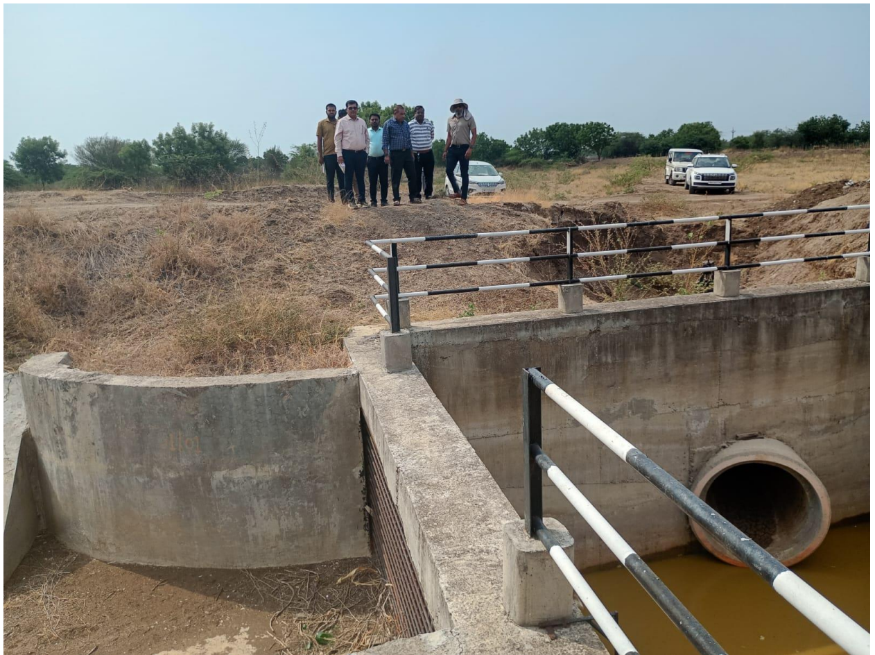
SBC main canal PDN starting chamber point at 85 km
