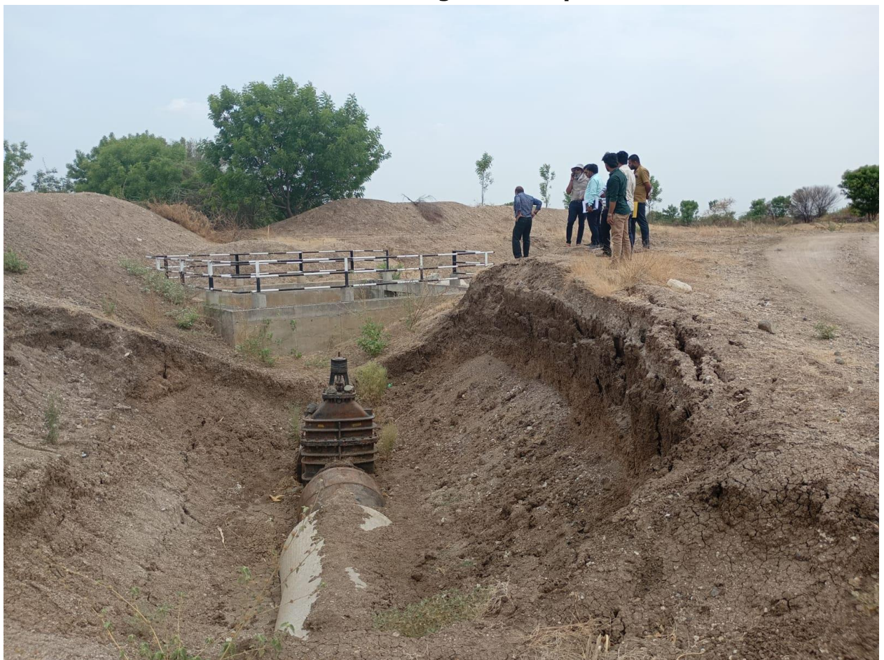
SBC main canal PDN starting point at 85 km
