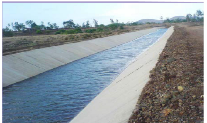
Figure 1 Right Main Canal
