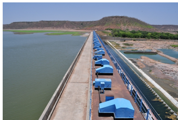
Mohini pick up weir I
