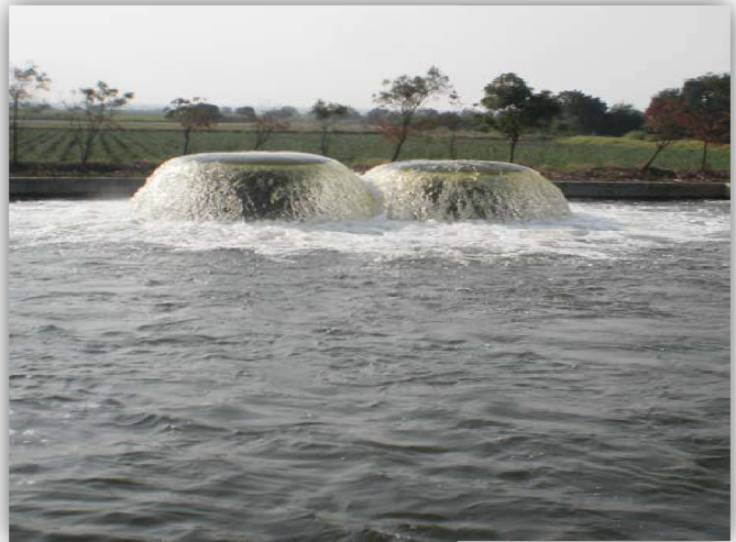
Balundagi Delivery Chamber
