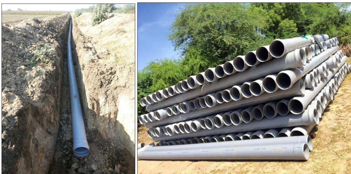
Laying & Stacking of PVC Pipes: Sokli U.G.P.L. Ta. Viramgam, Dist. Ahmedabad
